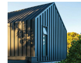
ENSEAM LYSAGHT ROOFING
