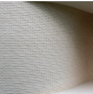
CURVED BRICKWORK WALLS
