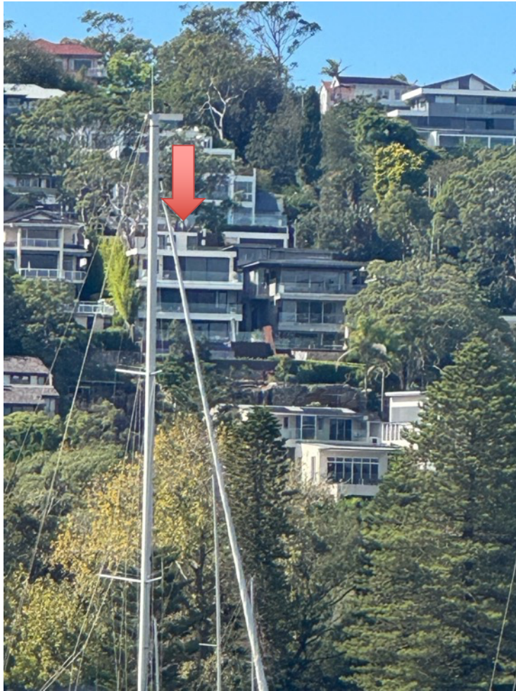
Figure 4 Viewpoint from the waterway to the subject site (max zoom)
