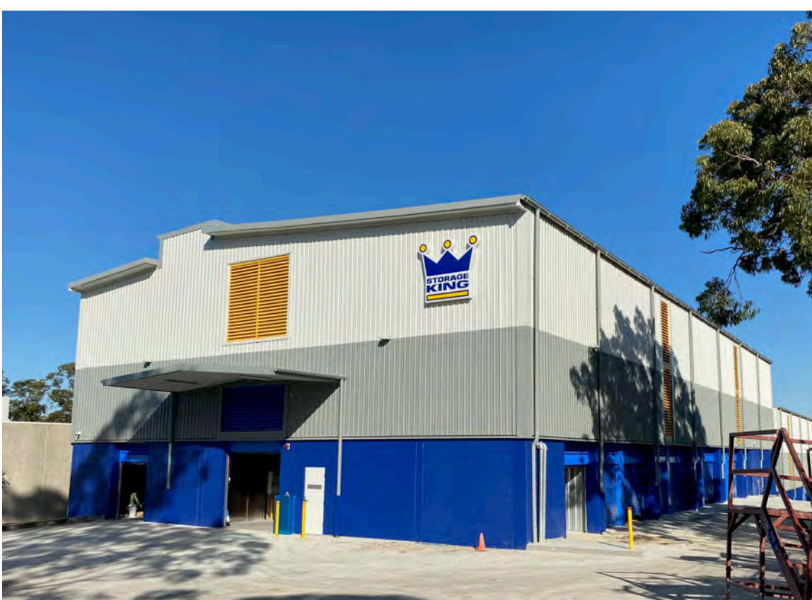
VIEW OF BUILDING 2 SHOWING EXISTING SIGNAGE
