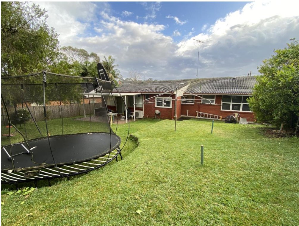
Figure 9: Looking north west the rear of the existing dwelling
