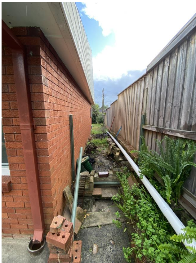
Figure 11: Looking north, the eastern side boundary of the existing dwelling
