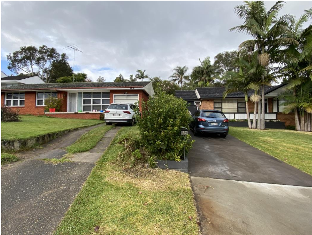
Figure 6: The existing dwelling and the immediate neighbour to the west at 27 Epping Drive (also showing the existing driveway access)
