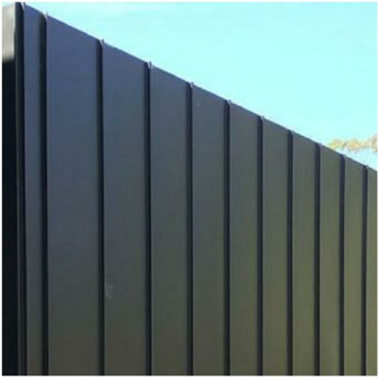
CLADDING - STANDING SEAM. COLOUR: DARK GREY
