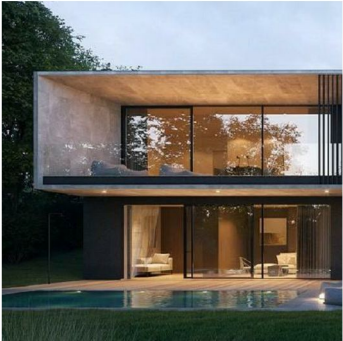
FEATURE WALL - OFF-FORM CONCRETE
