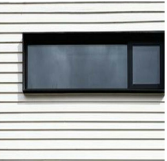
H - ALUMINIUM WINDOW FRAMES FINISH = DULUX RAKU
