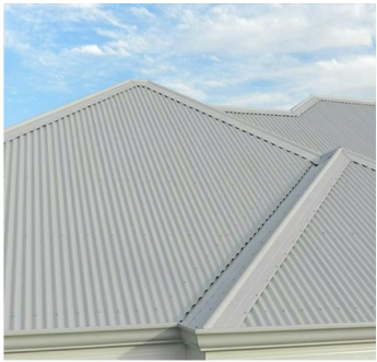
D - COLORBOND ROOFING FINISH = SHALE GREY
