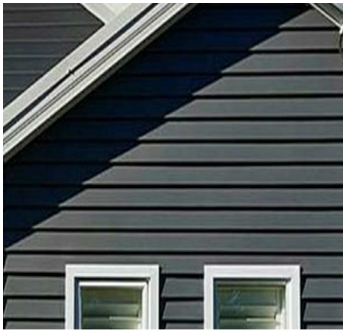
A - LINEA WEATHERBOARD FINISH = DULUX RAKU
