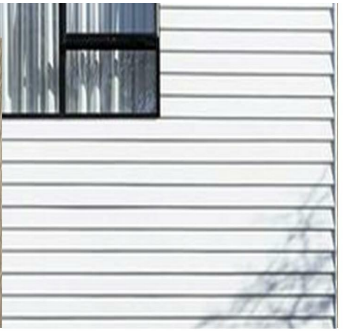
G - LINEA WEATHERBOARD FINISH = DULUX TERRACE WHITE
