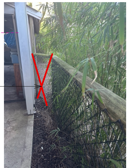
EXISTING SOUTH BOUNDARY FENCE AT GARAGE FRONT.
