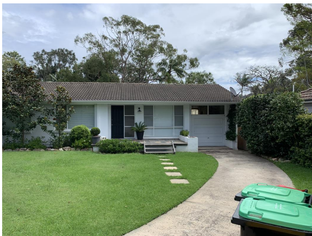
Fig 3: View of location of proposed carport forward of the existing dwelling, looking west from Burrawong Road
