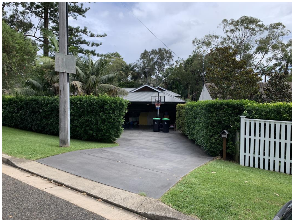
Fig 4: View of adjoining carport on a reduced front setback, looking west from Burrawong Road
