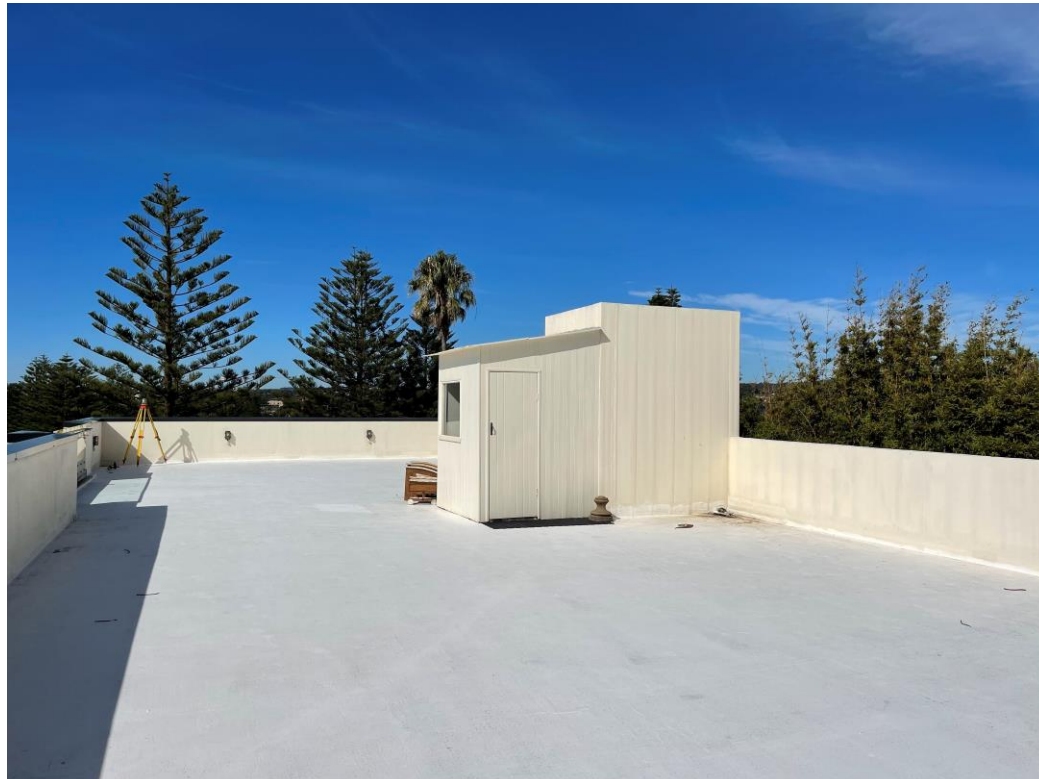
Fig 9: View of the existing roof top conditions, looking south
