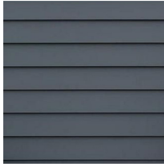
2. Weatherboard Cladding - 'Dulux Domino' Colour
