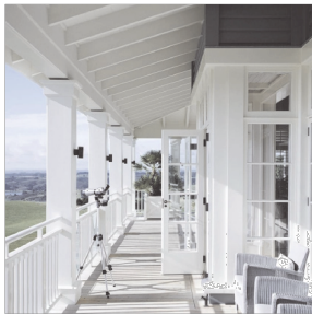
7. White Painted Timber Post, Beams & Eaves over External Areas
