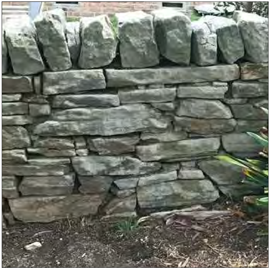
S - EXISTING STONE WALL
