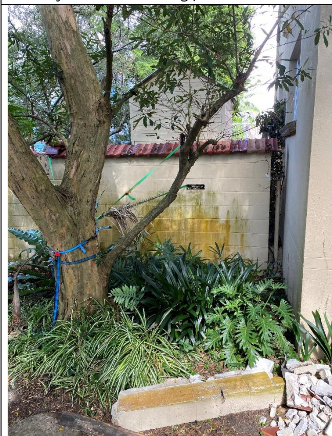
Proximity of Tree 4 to existing premises
