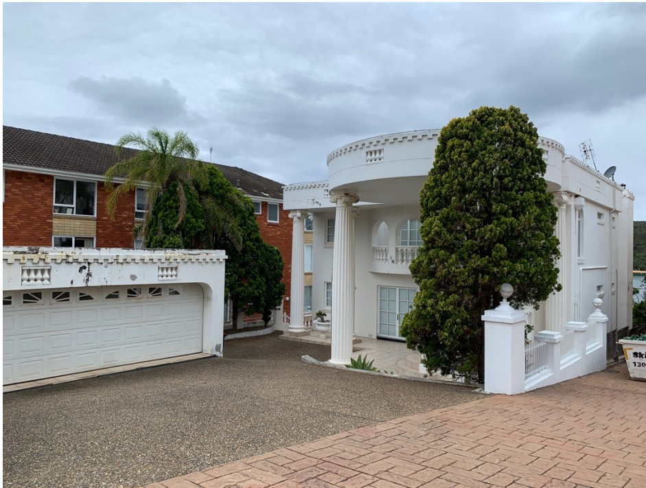
Photo 1 Overview of existing residence.
