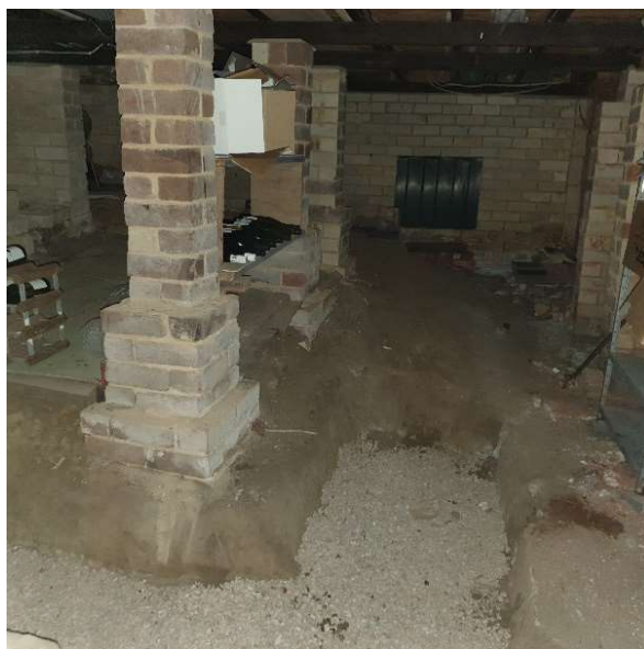
Photograph-6: Brick columns and walls supporting the site-dwelling. View looking east from below the site-dwelling.
