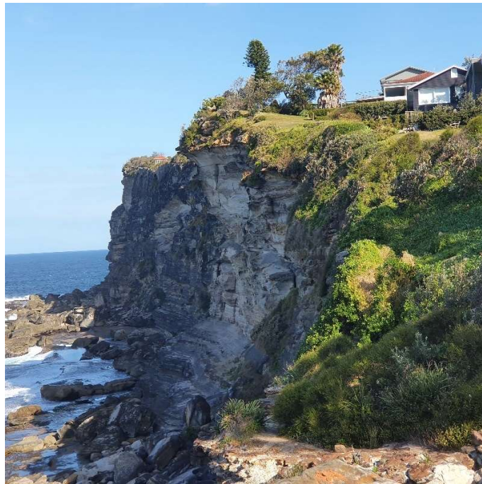
Photograph-5: Full cliff face located below the site. View looking south from Bangalley Park estimated height \geq 25\text{m}
