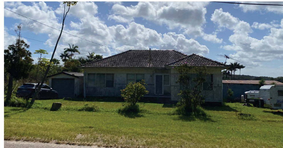
3 - Wilga Street - single storey dwellings on large lots with hipped roof form
