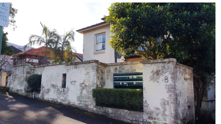
CONDITION OF FRONT FENCE
