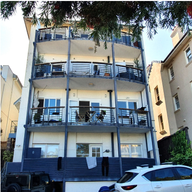
EAST ELEVATION. rear of building
