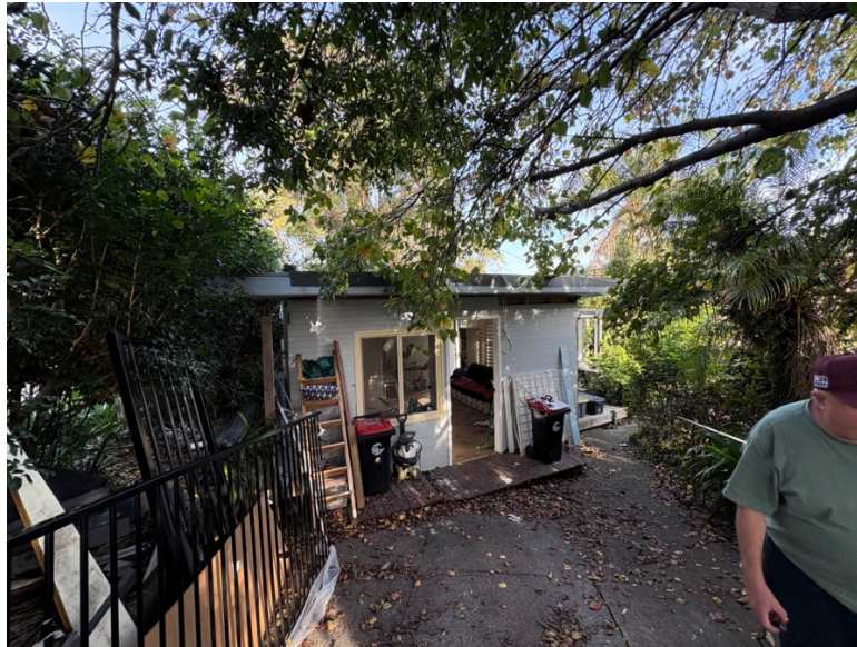
View of Existing Structure from Driveway
