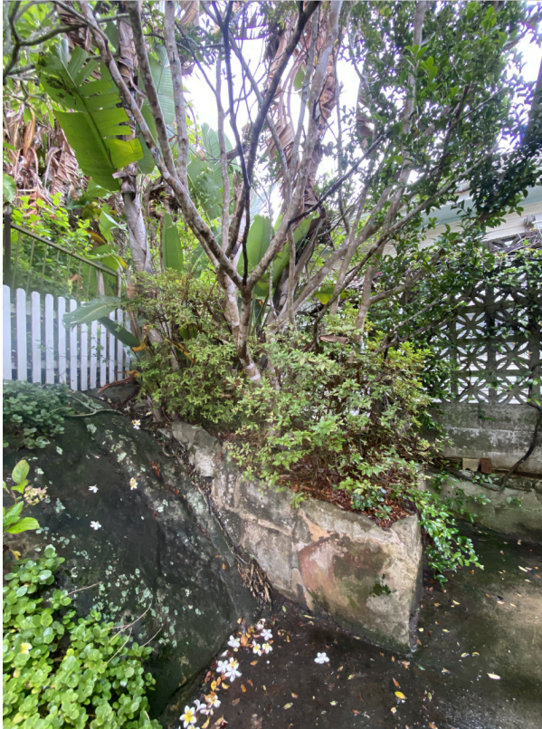
Figure 9: Site photo at rear of dwelling
