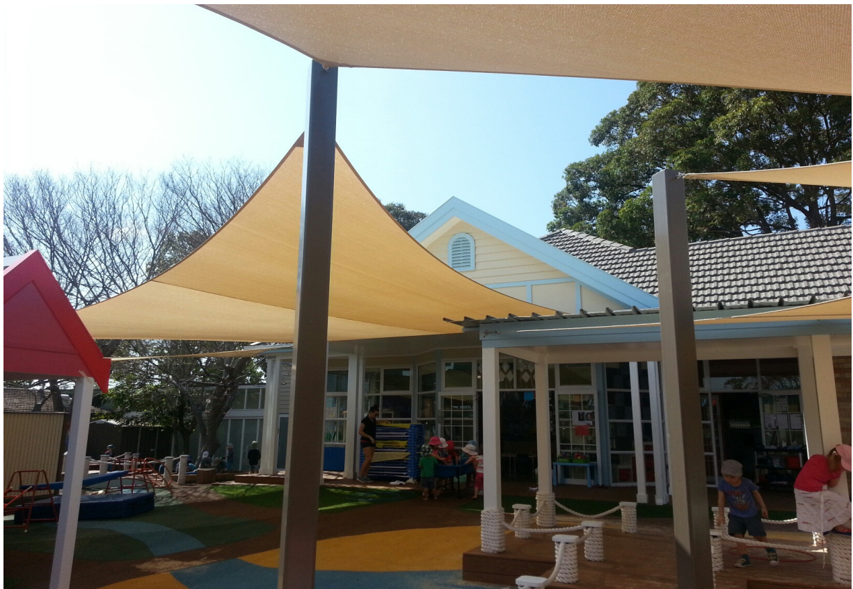
Photo No: 3 Example of low profile shade structure Little Diggers Preschool Veterans Parade, Collaroy
