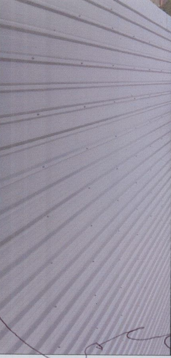
Non-Reflective metal roof (Mid Grey) sheathing to roof and light shelves Colorbond® or equivalent (Basic SA <0.475) on 5 pitch. All associated rainwater goods to match.
