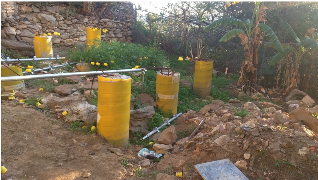
Photo 2: Pool piers. Pool is mainly supported above ground.
