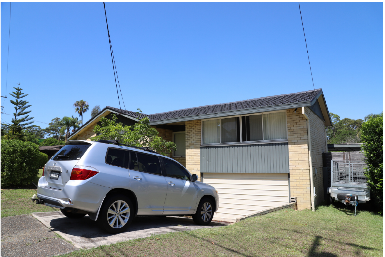
View from along Coora Avenue
