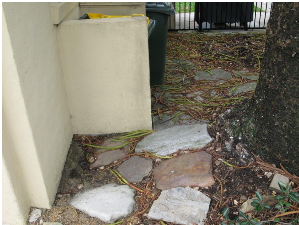
Figure 4: Illustrates tree trunk location & existing competing structures.
