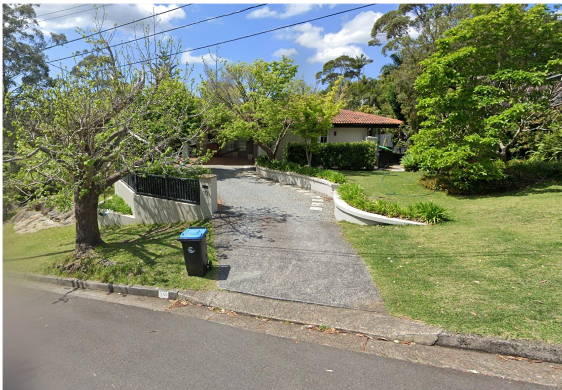
FIGURE 6: Street View, Rear – Secondary front setback-10 Spence Place Belrose. Source Google Maps. 9
