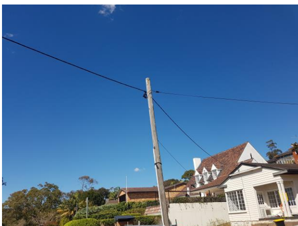
Above ground electrical supply
