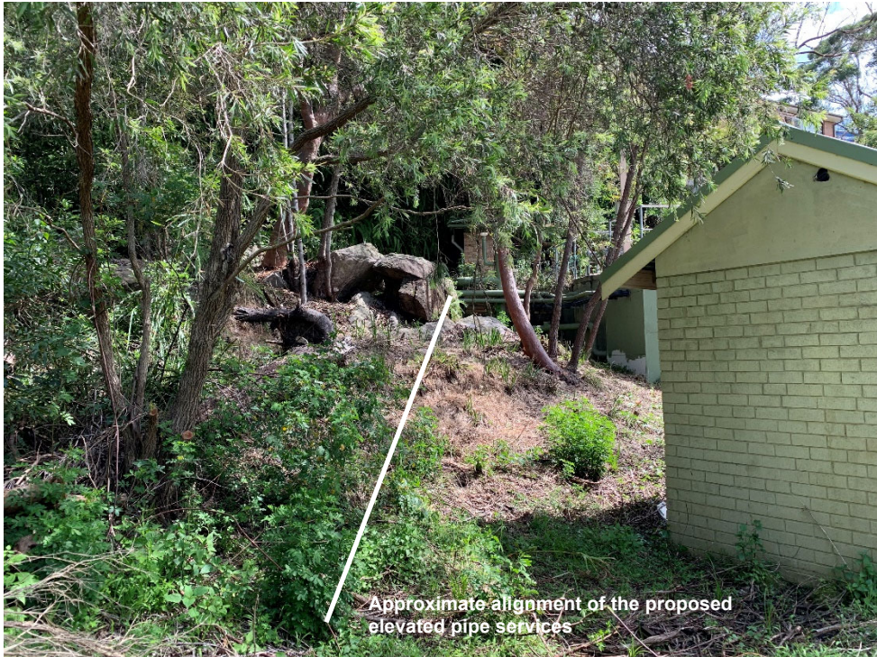
Figure 4.2 - View of the rocky terrain and the alignment of the proposed pipes which are to be elevated above ground and supported on piers.
