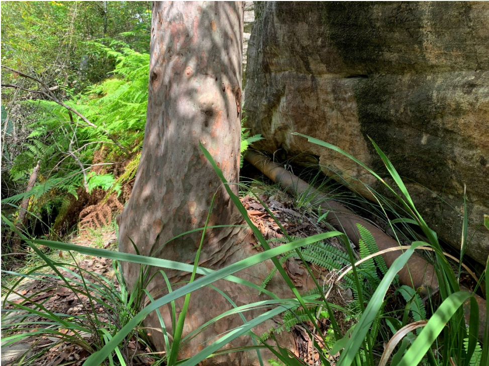
Figure 4.3 - The base of Tree No. 96.1 showing the existing cast iron rising sewer main (right).
