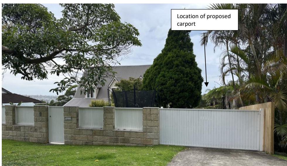
Figure 19: Views across the subject site, looking east.
