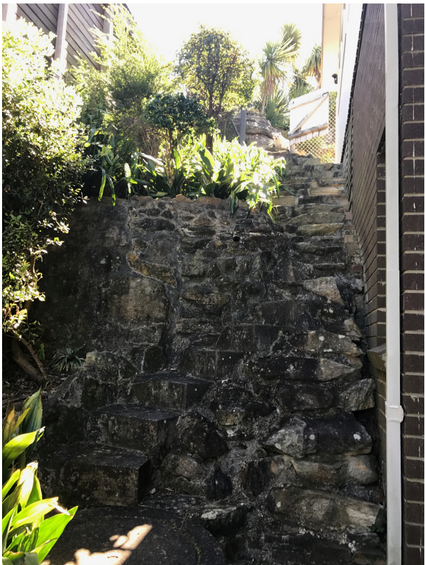
EXISTING WEST SIDE BOUNDARY STEPS
