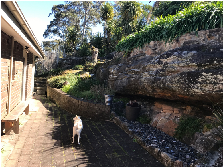
EXISTING REAR ROCK WALL
