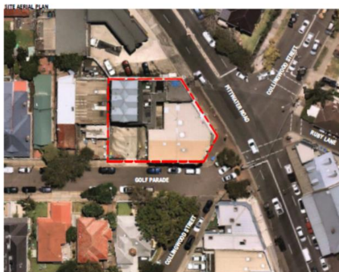
Above – Fig. 01 – Aerial photo of Site in Pittwater Road with vehicle access off Golf Parade
