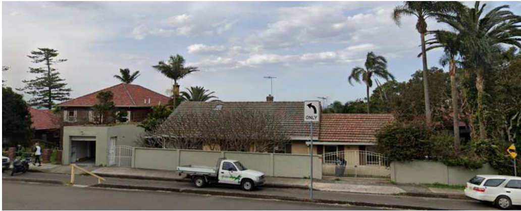
Figure 58: The site No.35 Reddall Street, Manly.
