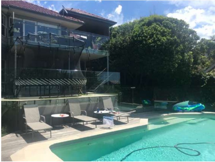
Figure 16: View from rear yard up to dwelling at No. 29 Reddall Street, Manly.
