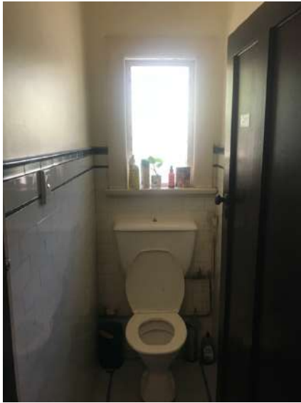
Figure 54: First floor WC., No. 31 Reddall Street, Manly.
