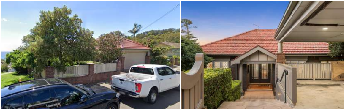
Figure 25 and 26: The site No. 29 Reddall Street, Manly, viewed from Reddall Street.
