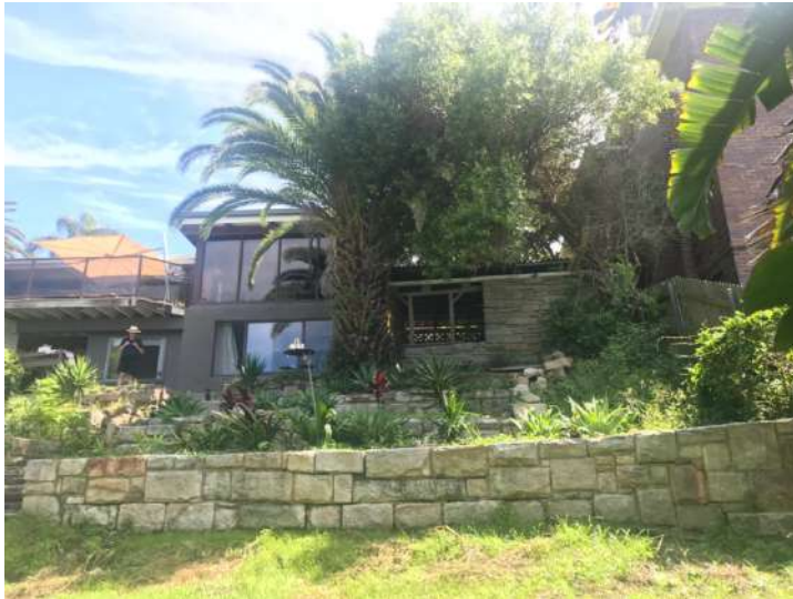
Figure 22: View from rear yard up to No.35 Reddall Street.
