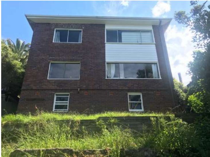
Figure 17: View from rear yard to dwelling at No. 31 Reddall Street, Manly.
