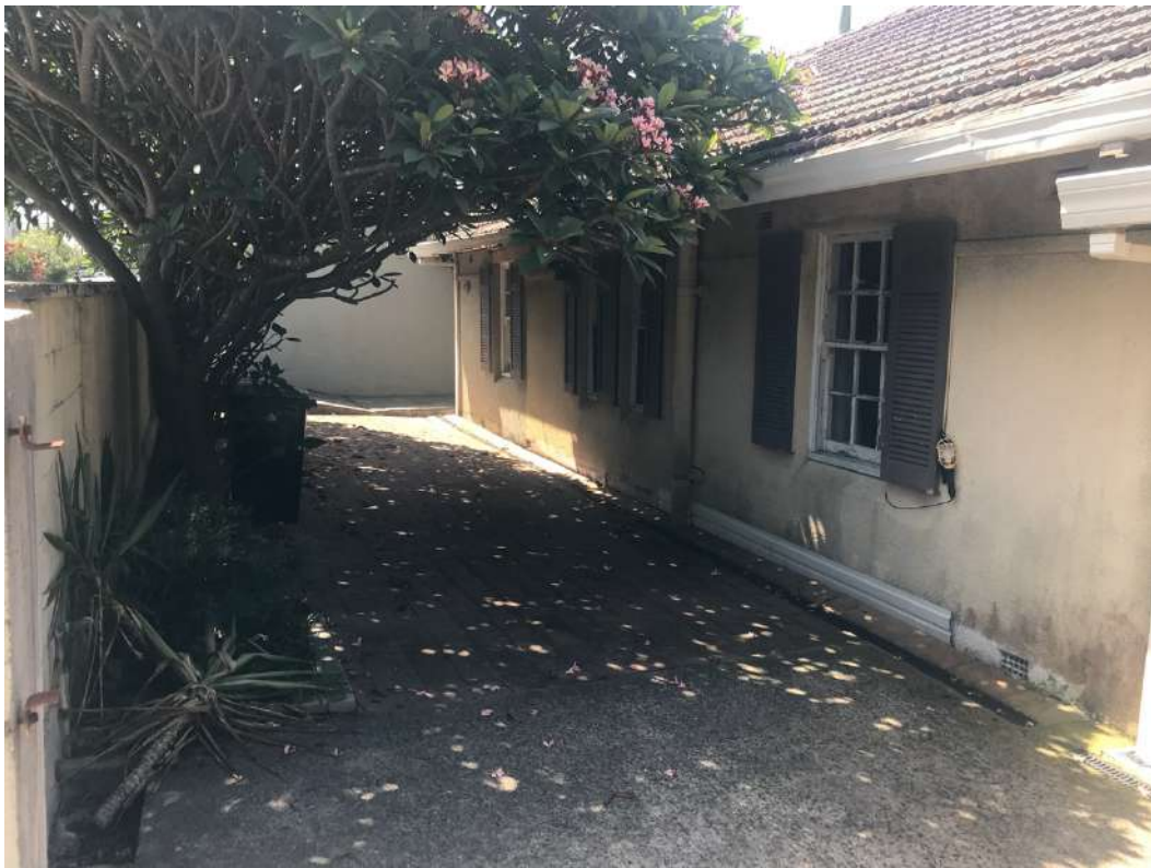
Figure 61: The front yard, No.35 Reddall Street, Manly.
