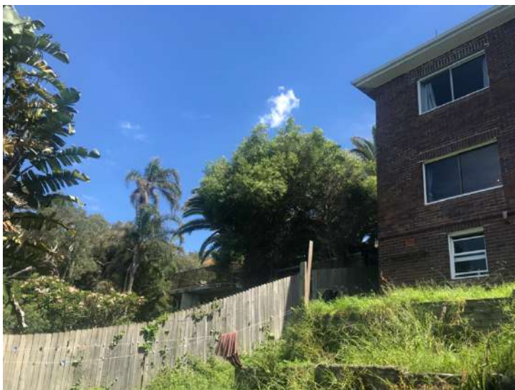
Figure 18: View from rear yard toward dwelling at No. 35 Reddall Street, Manly.
