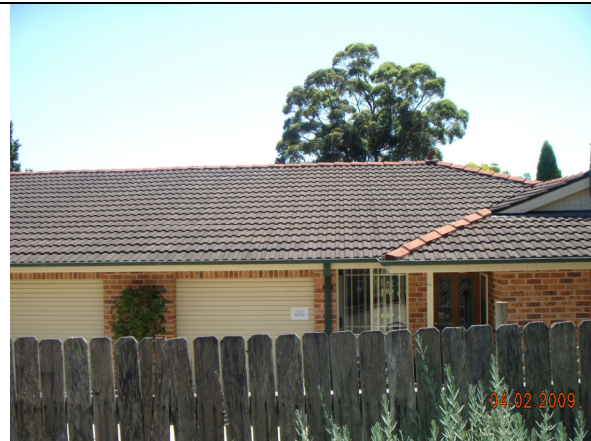
Picture taken at the approximate level of the proposed deck extension, looking north at No's 322 A and 333 B Warringah Road..
