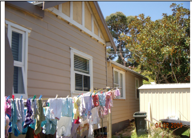
The location of the proposed addition for the ensuite. Picture taken looking south.
