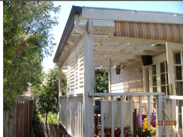
The existing rear deck to be extended. Picture taken looking east.
