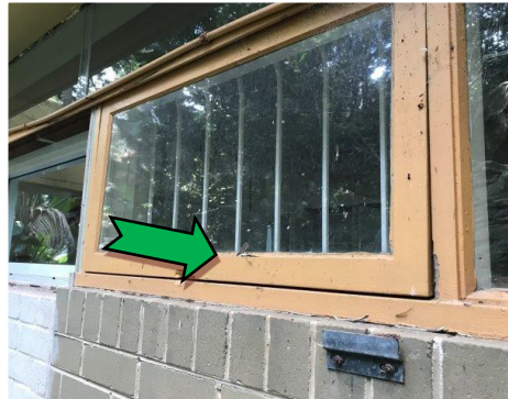
4. Exterior, south-west corner of building, window frame – non asbestos-containing window mastic.
