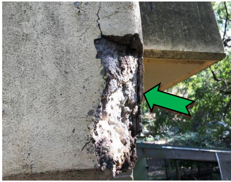
1. Exterior, north-east corner of building – non asbestos-containing render finish to roof slab.
