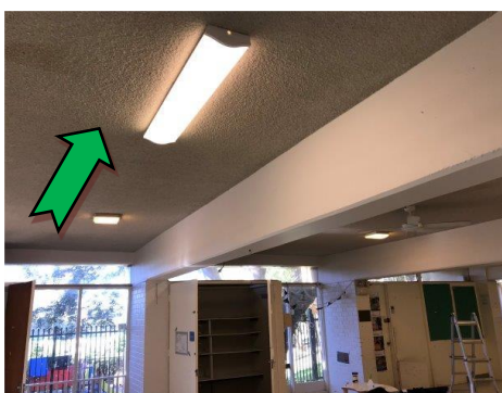
6. Interior, north section of playroom, ceiling – non asbestos-containing sprayed vermiculite.
