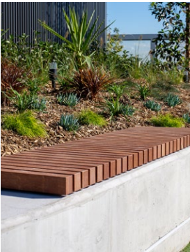
SW: insitu concrete class 2 with timber seating battens and led light strip
