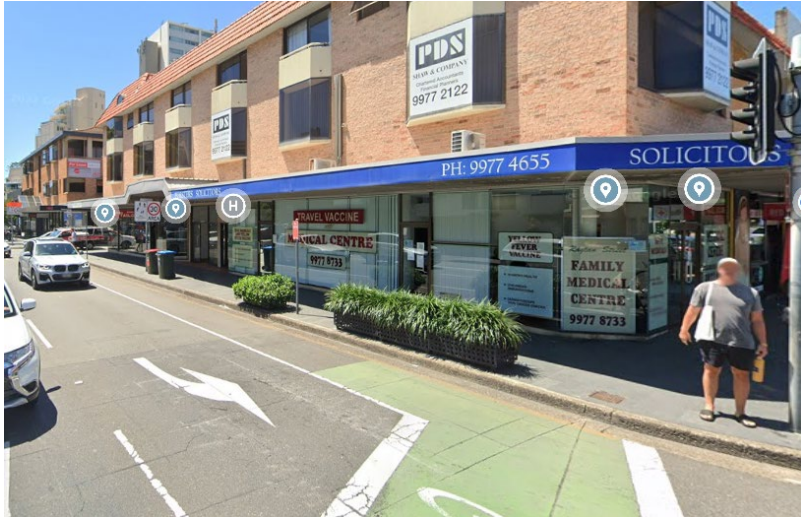
Lack of retail spill-out on street
