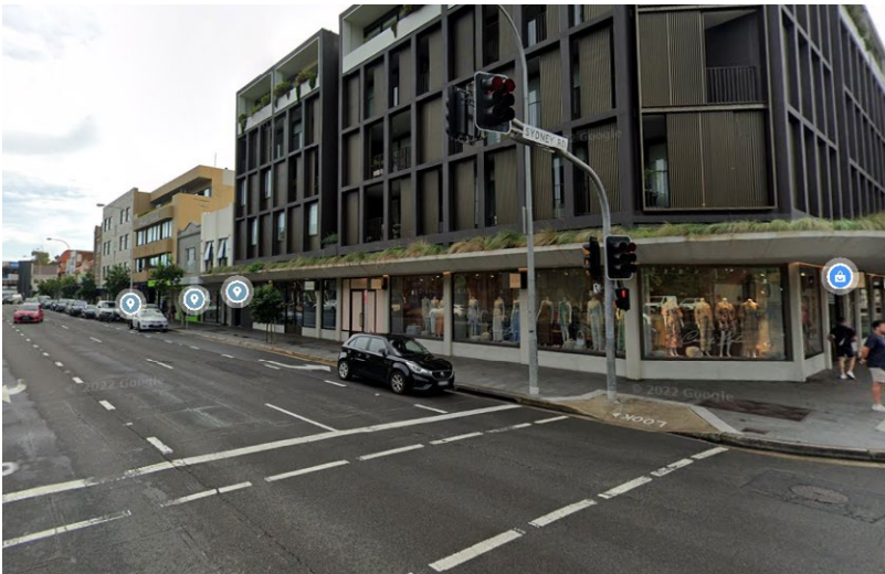
Green awnings supported
