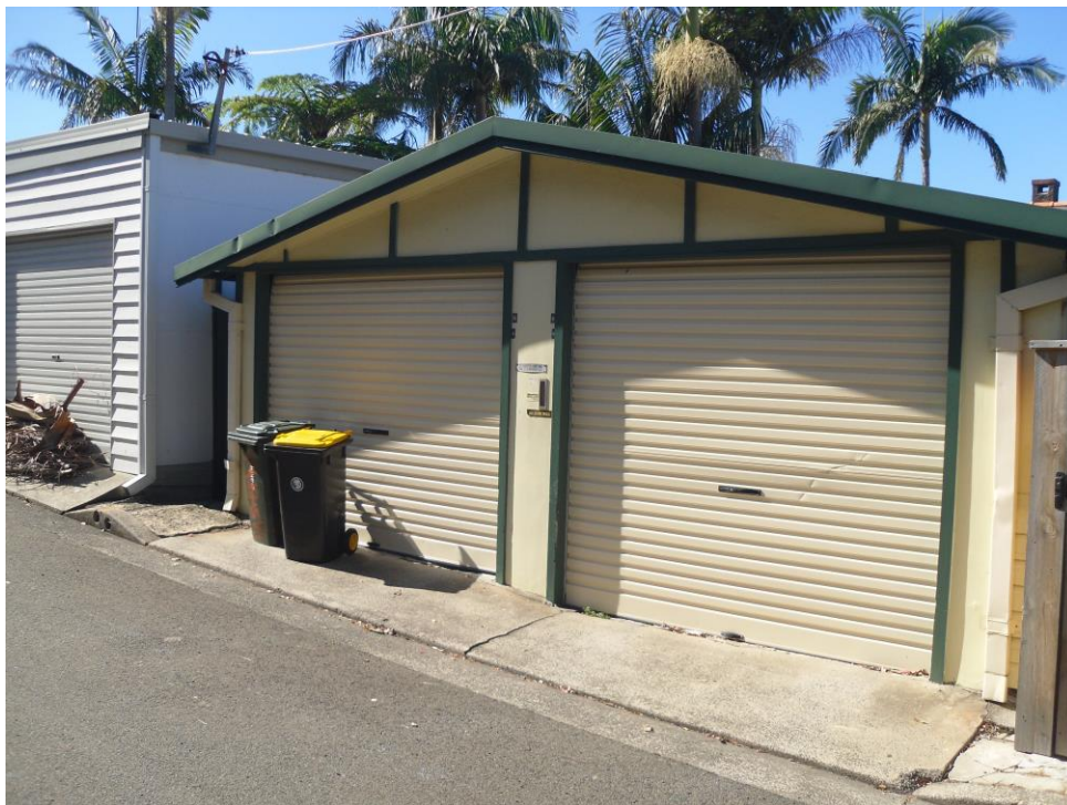
Fig 2: View of existing double garage building, looking north-east from Augusta Lane
