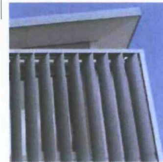
LV: Aluminium louvre blades, clear anodised finish. Louvretec pivoting "Maxi Louvre" or similar to match
