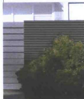
CB: Boral Designer block in "Charcoal", 90mm high with raked horizontal joints for front fence
