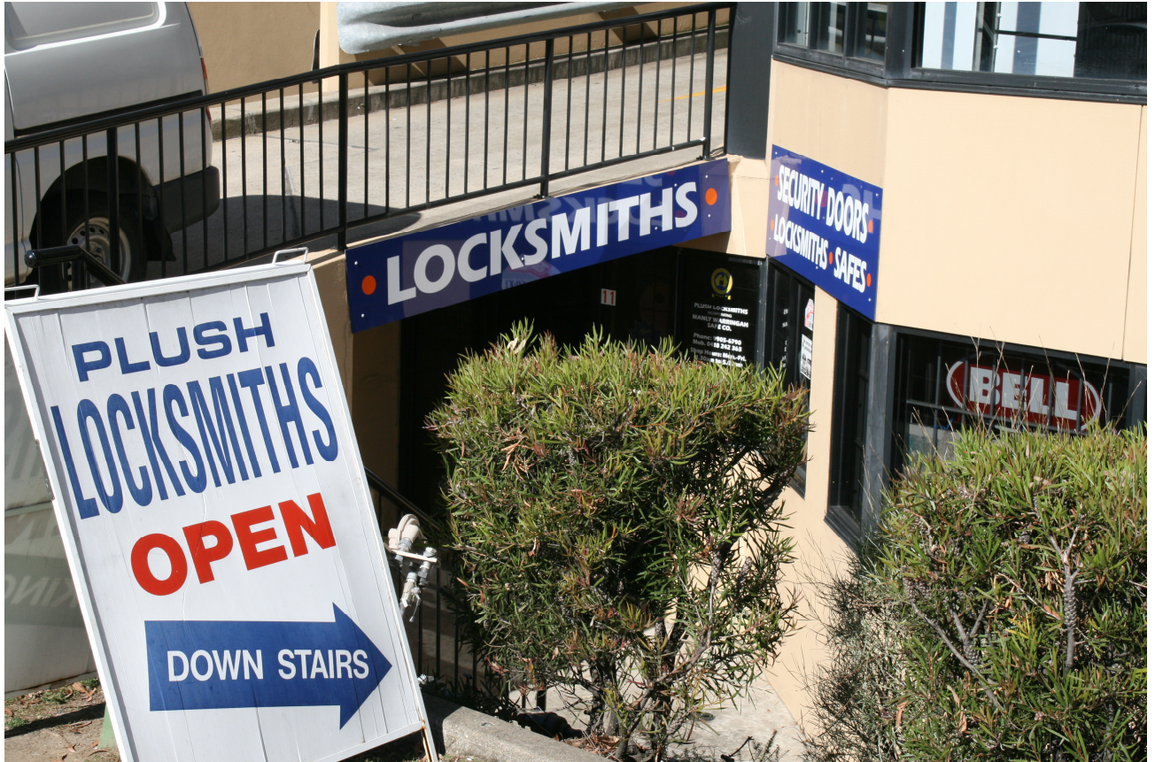
Photograph No:1 Original open landscaped area and open stair access to Lot 11. Lot 11 visible from the street footpath & signage from Pittwater Road.
