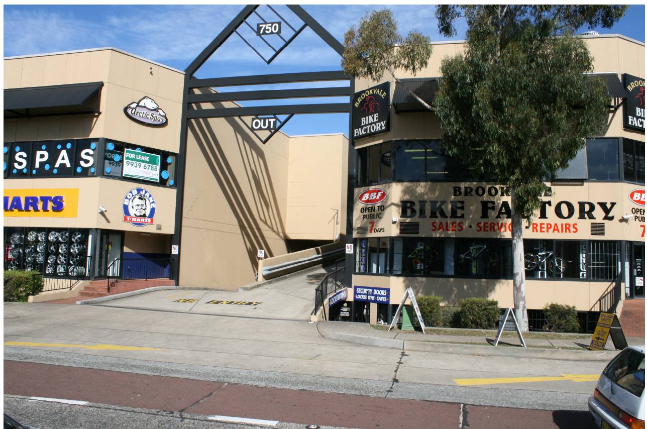
Photo No: 2 Original Landscaping which has been removed without consent including Significant tree planting
