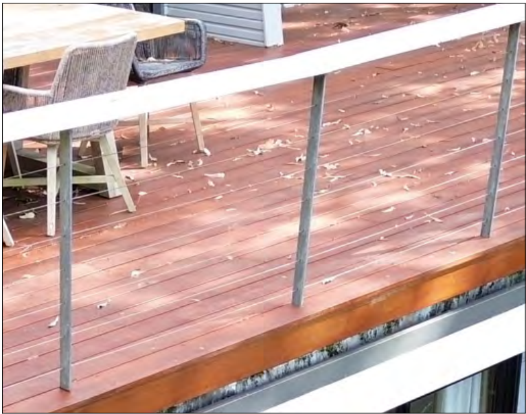
02 - EXTERNAL WIRE HANDRAIL TO MATCH EXISTING
