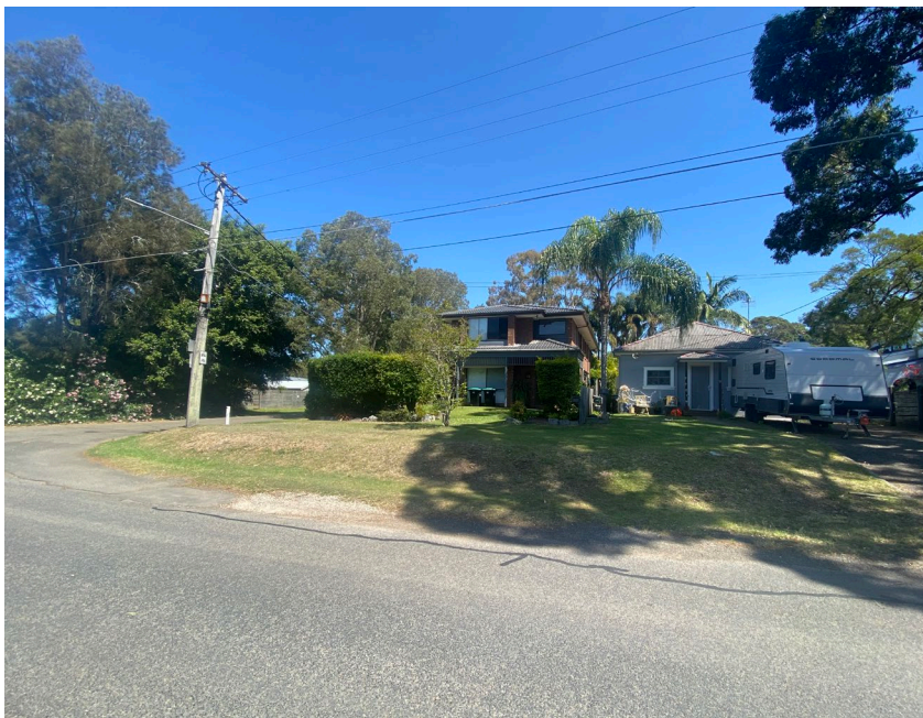
Raised Corner allotment of 15 and 17 Narroy Road, North Narrabeen (Photo facing South)
