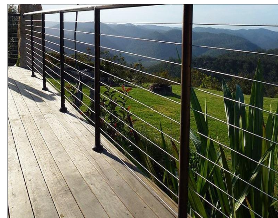
all balustrades rendered blockwork steel wire balustrade
