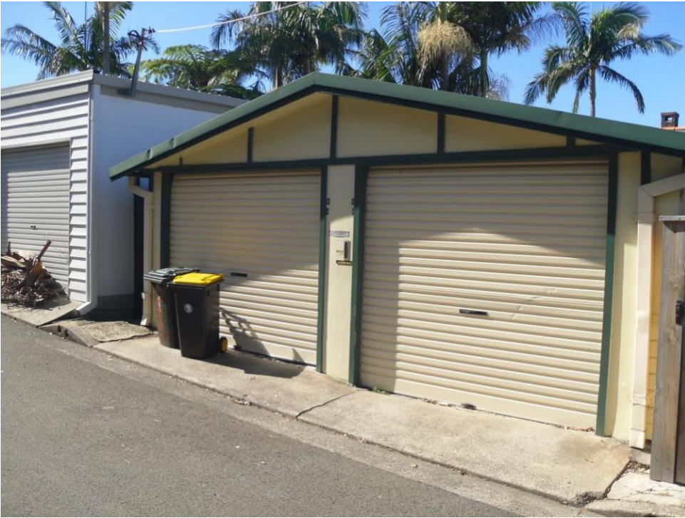
IMAGE 01: View of existing garage, facing Augusta Lane
