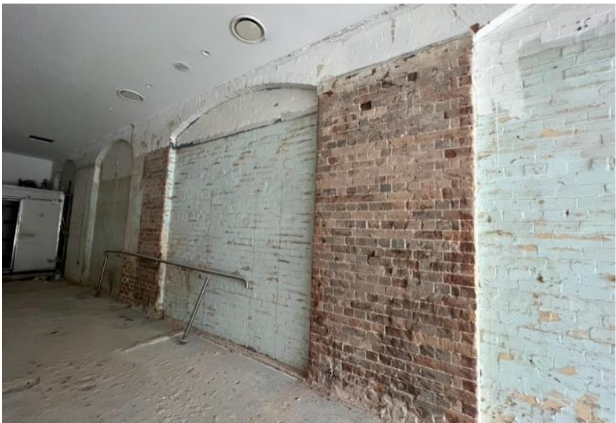
Figure 19 – Western wall of shopfront unit (Source: 3+1 Heritage, 2023)
