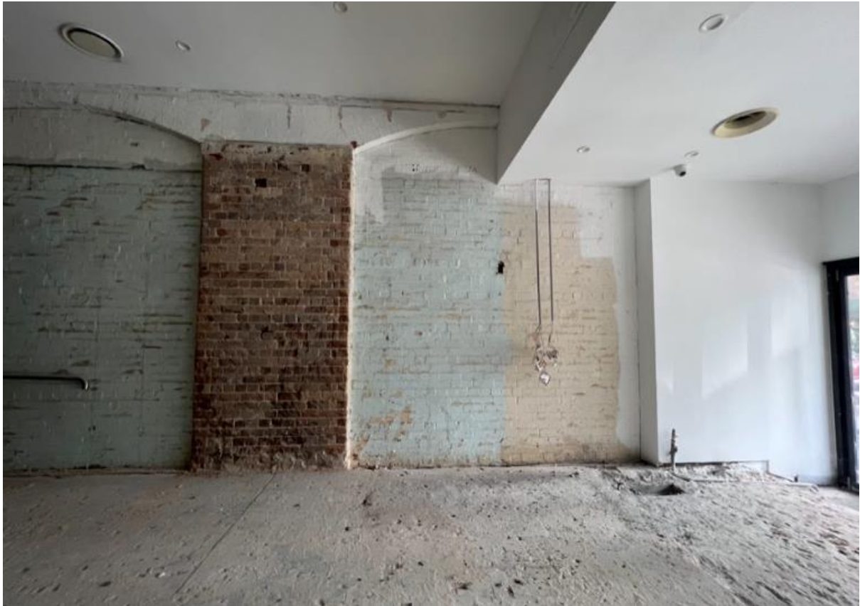
Figure 18 – Western wall of shopfront unit, including remnant archways and modern bulkhead (Source: 3+1 Heritage, 2023)
