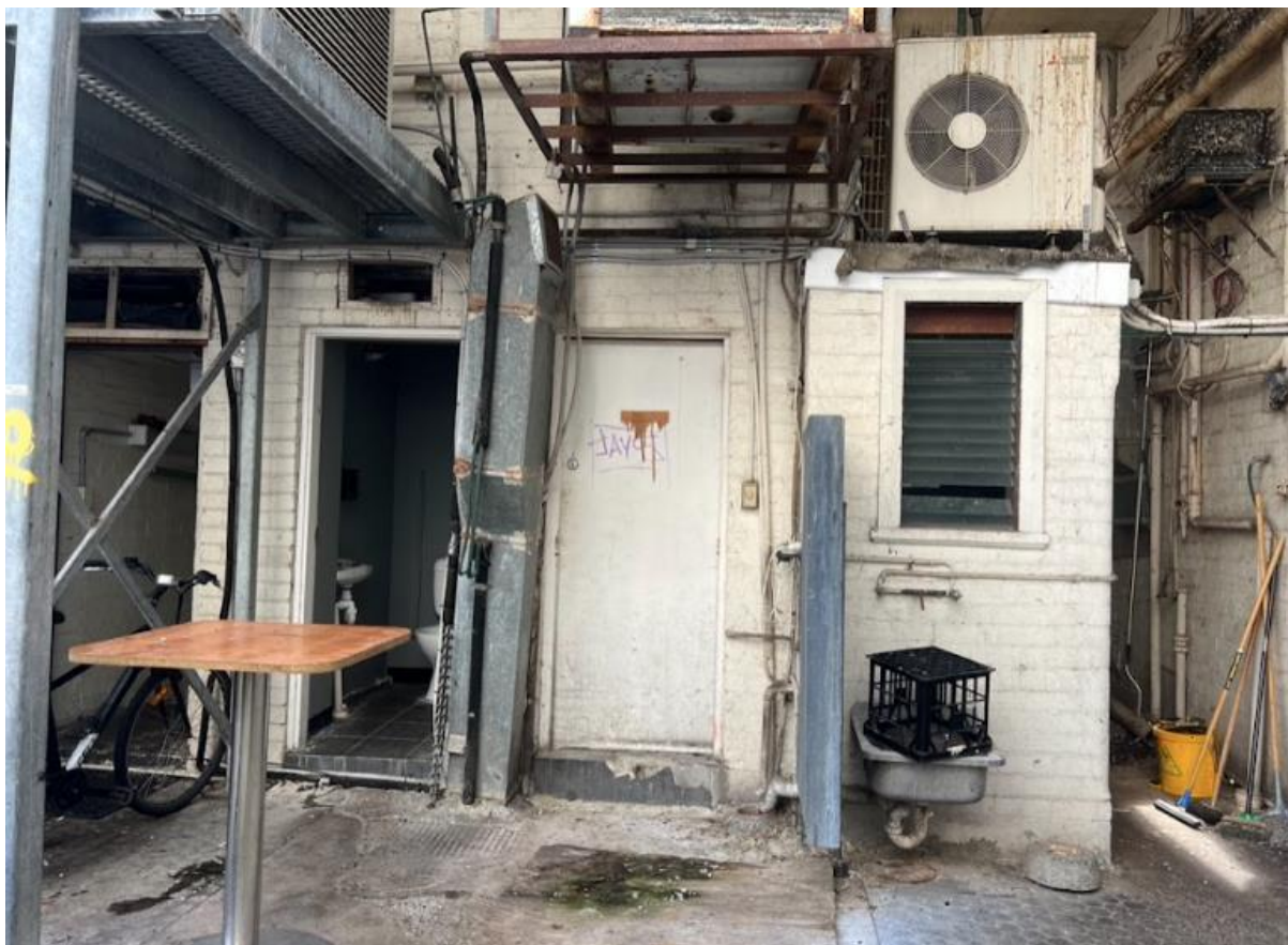
Figure 27 - Rear entrance and rear WC (Source: 3+1 Heritage, 2023)
