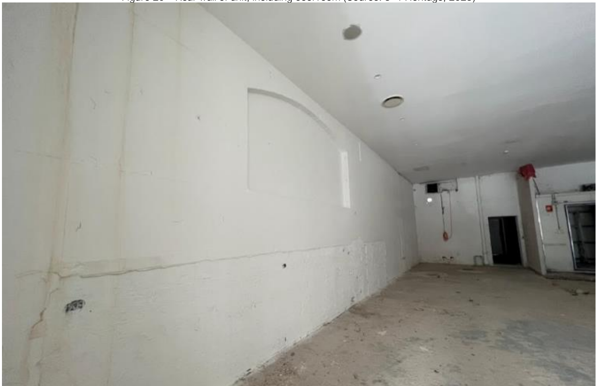
Figure 21 - Eastern wall of shopfront unit (Source: 3+1 Heritage, 2023)
