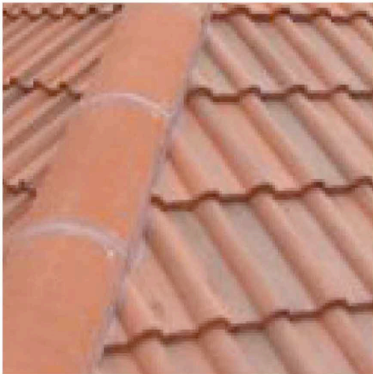
1. Existing roof tile.
