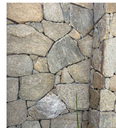
RETAINING WALL: LIGHT STONE
