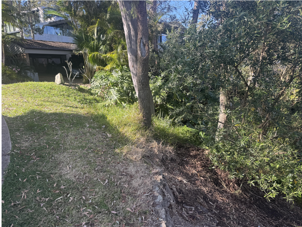
View of slope crest at Lisa Place
