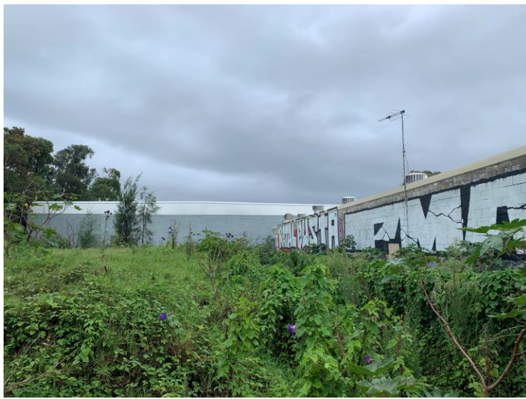
Photograph 7: Western portion of the site, looking south. Embankment sloping west with a gradient of approx. 1:1. Dense vegetation cover.
