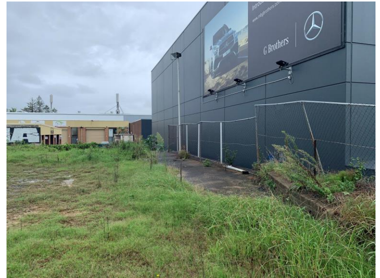
Photograph 6: Northern portion of the site, looking west.
