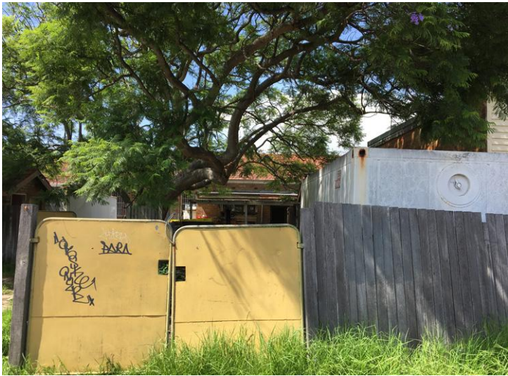
NO 62 MAY ROAD (THE SITE)
