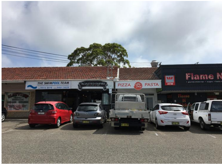
NO 54-52 MAY ROAD (THE SITE)
