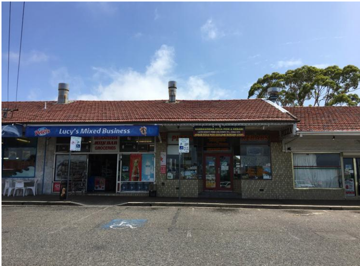
NO 60 MAY ROAD (THE SITE)
