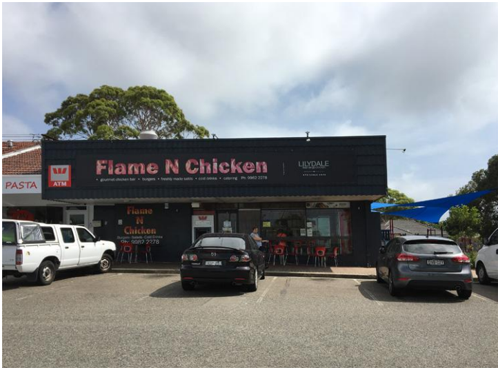
NO 54-52 MAY ROAD (THE SITE)
