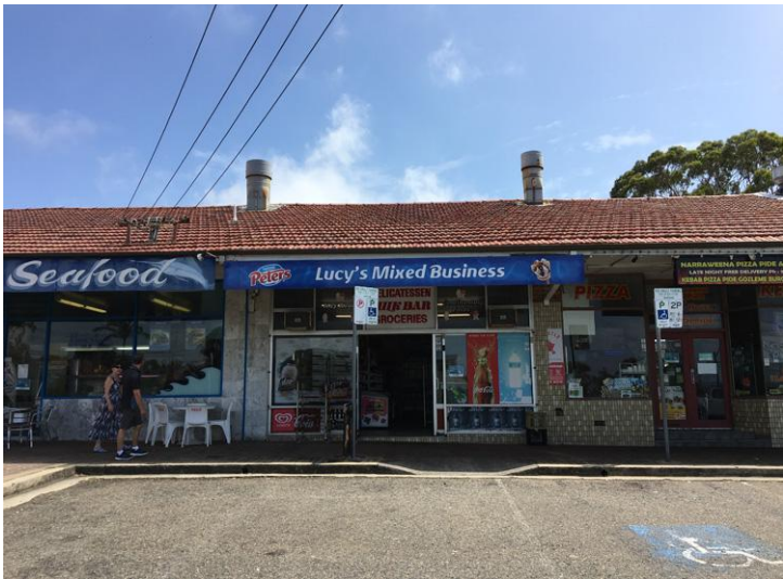
NO 62 MAY ROAD (THE SITE)
