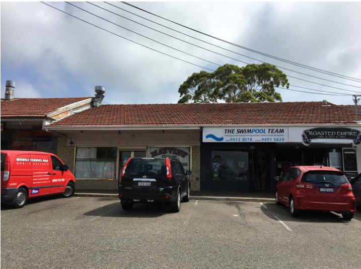
NO 58-56 MAY ROAD (THE SITE)
