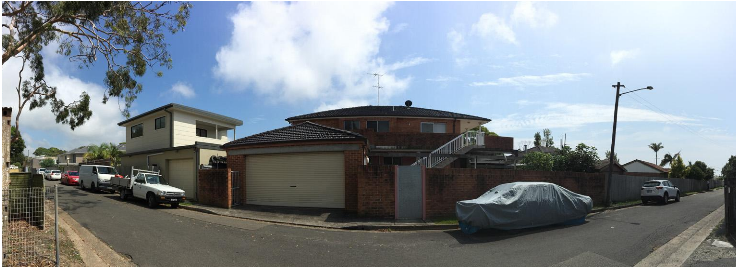
08 NORTHERN VIEW FROM NO 52 MAY ROAD (THE SITE)
