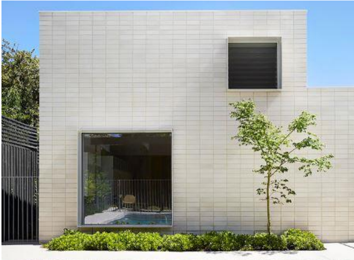
ALU 2 ALUMINIUM - WINDOW/BALCONY SURROUND FINISH SIM/EQ. TO DULUX POWDERCOAT 'OFF WHITE'
