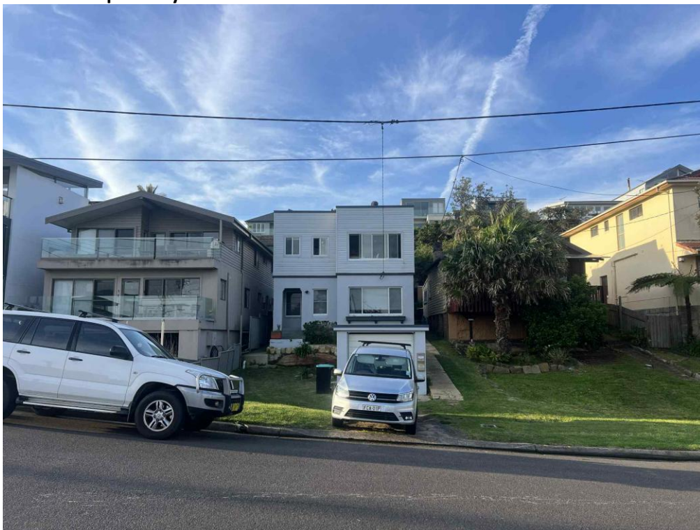
Photograph of the Site – 46 Pitt Road, North Curl Curl
