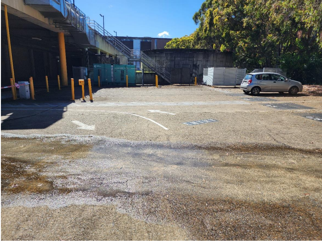
Photo 1 - General Site Photo Facing East at CBH01
