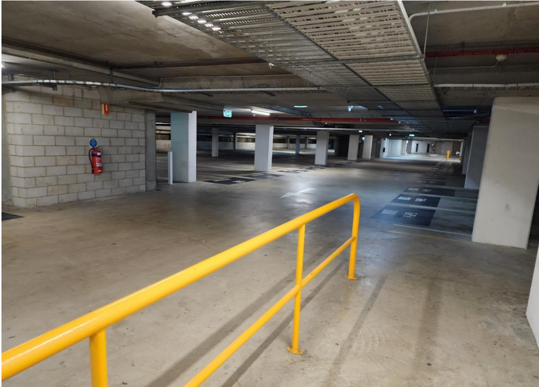
Photo 5 - Existing Basements Level 1 of 2
