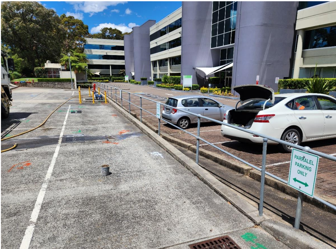
Photo 4 - General Site Photo Facing East at CBH02
