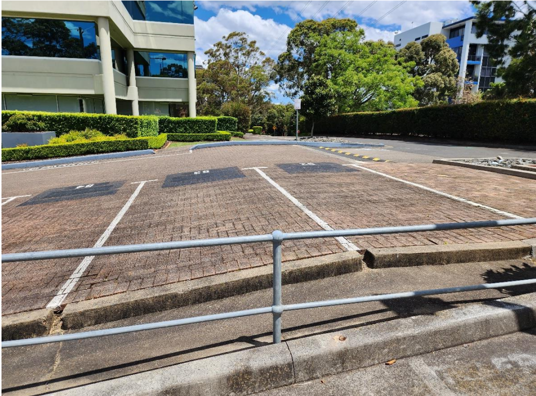
Photo 3 - General Site Photo Facing South at CBH02
