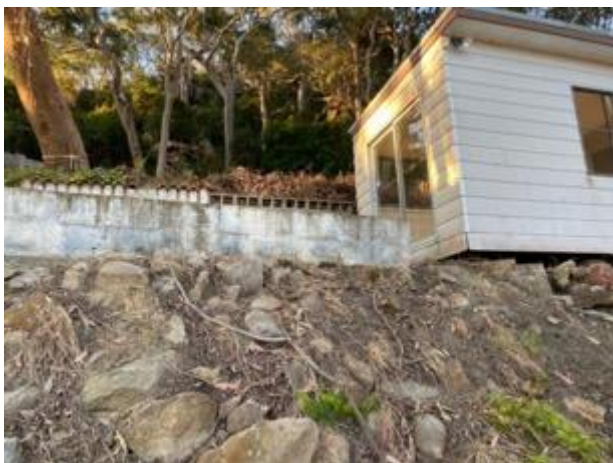
Plate 3. Granny flat and existing retaining walls in the area of the proposed pool
